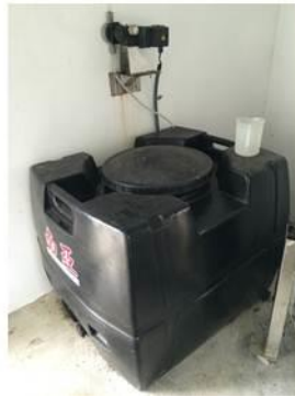
Drinking water filtration and chlorination disinfection equipment
