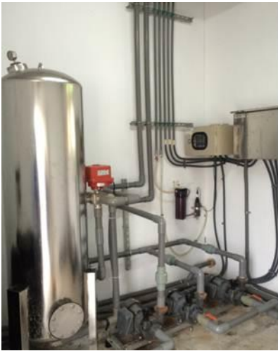
Drinking water filtration and chlorination disinfection equipment
